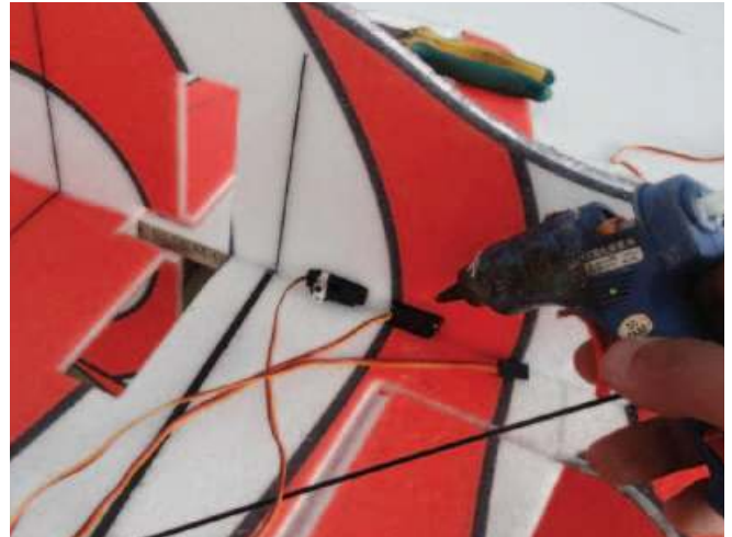
Same way to install fuselage's servos. Let the 2 servo's wires in same side.
